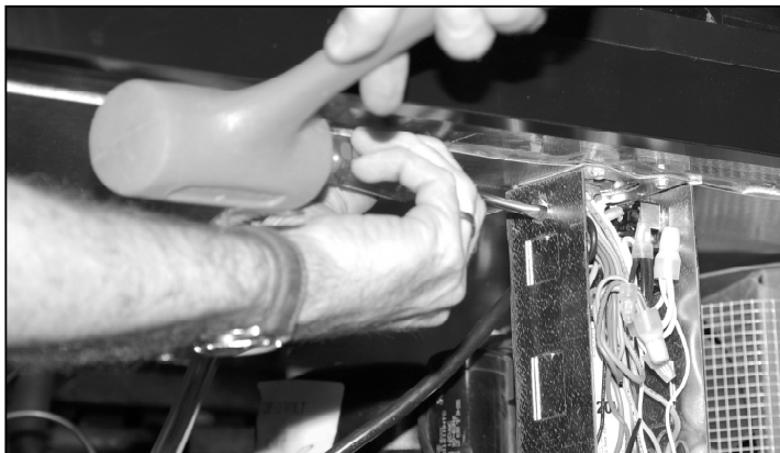
Figure 3. Driving out knockout
